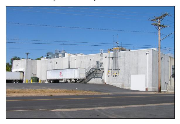
Limited site area along with the need for durability dictated the use of precast concrete for this 9800 sq. ft. spiral freezer building addition. Precast double—tees were used for the upper floor & roof while insulated precast concrete flat panels were used for the walls. Below grade concrete retaining walls were cast in place.
