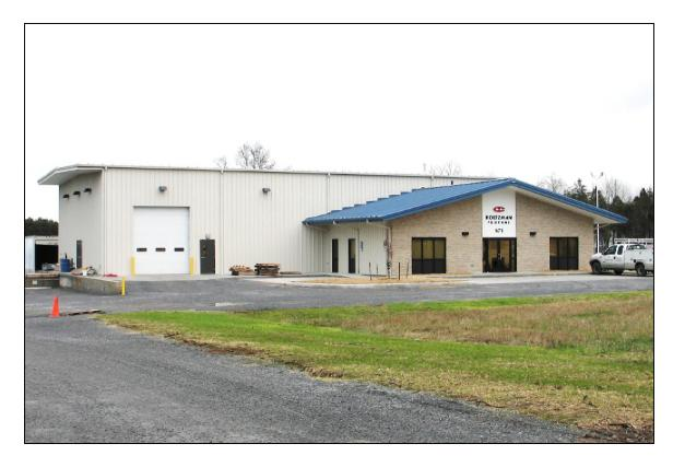
This 6500 sq. ft. building provides warehouse, office and showroom space for Holtzman Propane, LC. Two different pre—engineered metal building profiles were used to create a 12 foot high office wing and 22 foot high warehouse wing.
