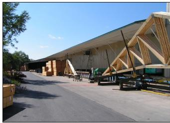
This project involved the adaptive reuse of an old outdoor crane rail structure into a new truss manufacturing facility. New roof trusses and metal wall panels were added to enclose the 26,000 sq. ft. space. The company manufactures wood floor and roof trusses, providing services throughout the Shenandoah Valley.
