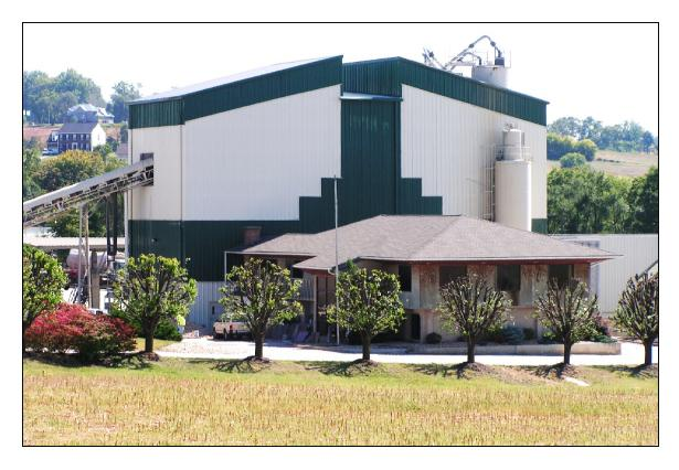
This 57 foot tall structure provides a complimentary backdrop to the existing concrete manufacturing facilities, while accommodating the need for an interior environment to keep concrete batch operations running uninhibited from the weather. Although removing the "industrial look" of a concrete batch plant may seem challenging, we were able to achieve an aesthetically pleasing solution by using decorative wall panels and a sloped roof.
