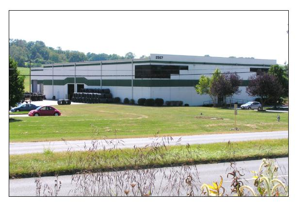
This 33,000 sq. ft. state—of—the—art reinforcing steel fabrication facility is constructed of tilt—up concrete wall panels & longspan open web steel joists. The wall panels provide a durable, yet aesthetically pleasing, exterior envelope, while the long span joists allowed for a clear span roof, enabling total flexibility in manufacturing operations.
